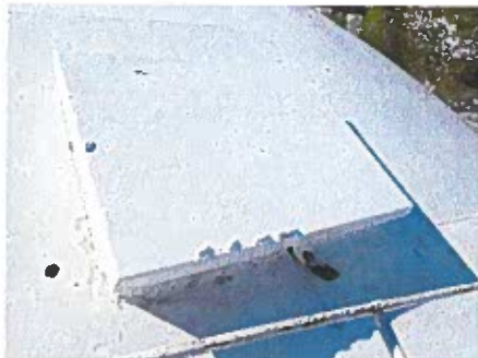
ACCESS HATCH PROTECTION
